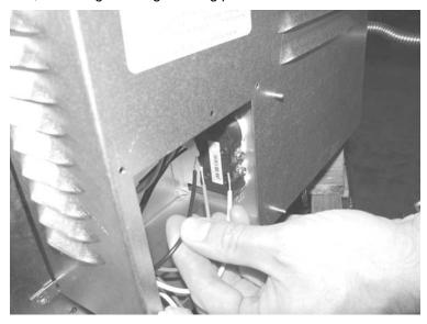
3. Remove the cover box from the fireplace. Attach the snap disk harness to the molex connector attached in step 1.
